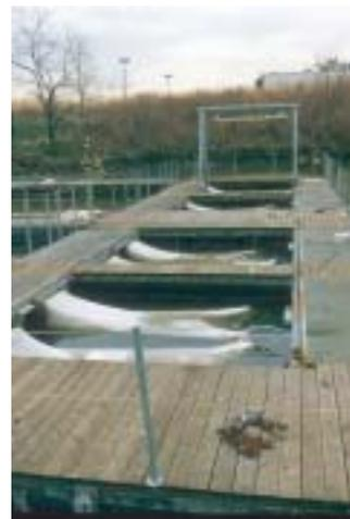
**Figure 3.26** New York City's use of end-of-pipe TrashTrap systems.
