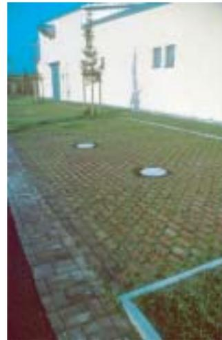
**Figure 3.14** Paver blocks for on-site infiltration in Essen, Germany.
