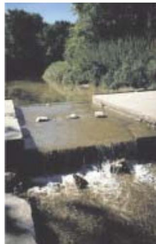
**Figure 3.10** Small drop structure obstruction in Lincoln Creek, Milwaukee, WI.
