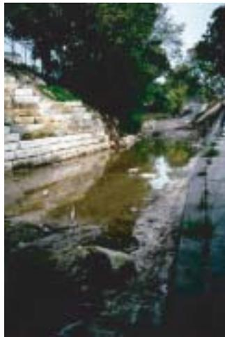
**Figure 3.8** Lined embankment along Waller Creek, Austin, TX.
